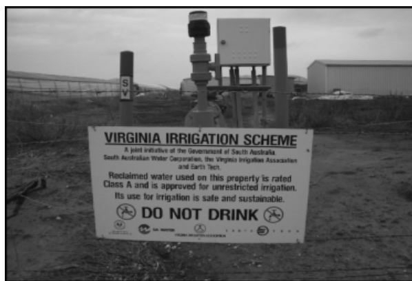
Fig. 4. Lilac pipes and sign board display used in the Virginia Pipeline Scheme.
